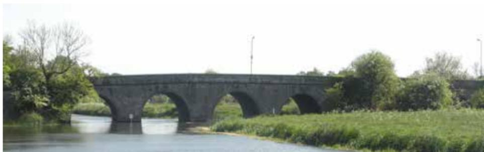
The Grade II listed bridge currently has a 13 tonne carrying capacity per vehicle. The 3 tonne limit will mean that large vehicles, including double decker buses, will not be able to use the bridge.
