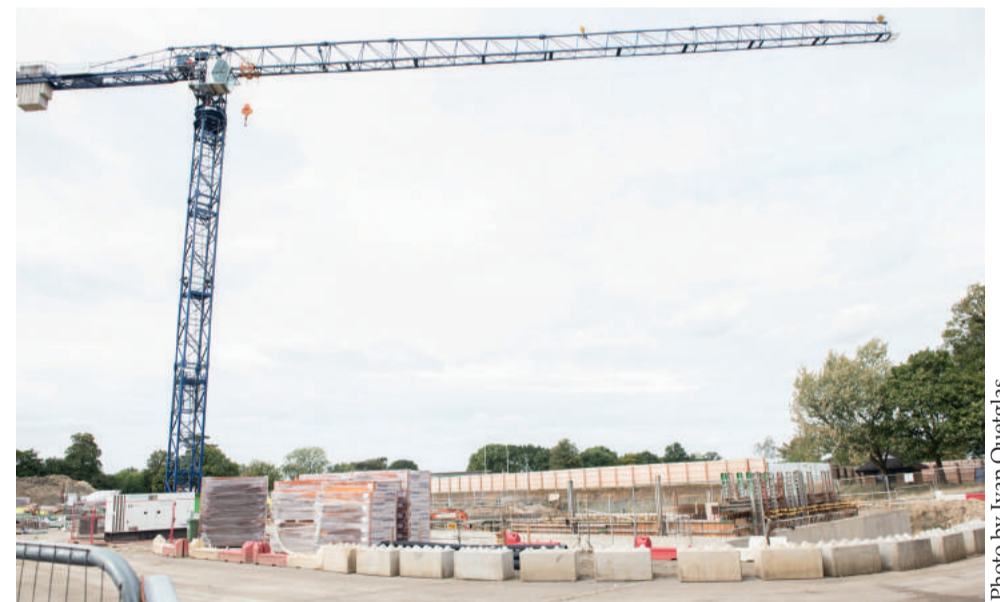
Construction work in November saw completion of the pool box
